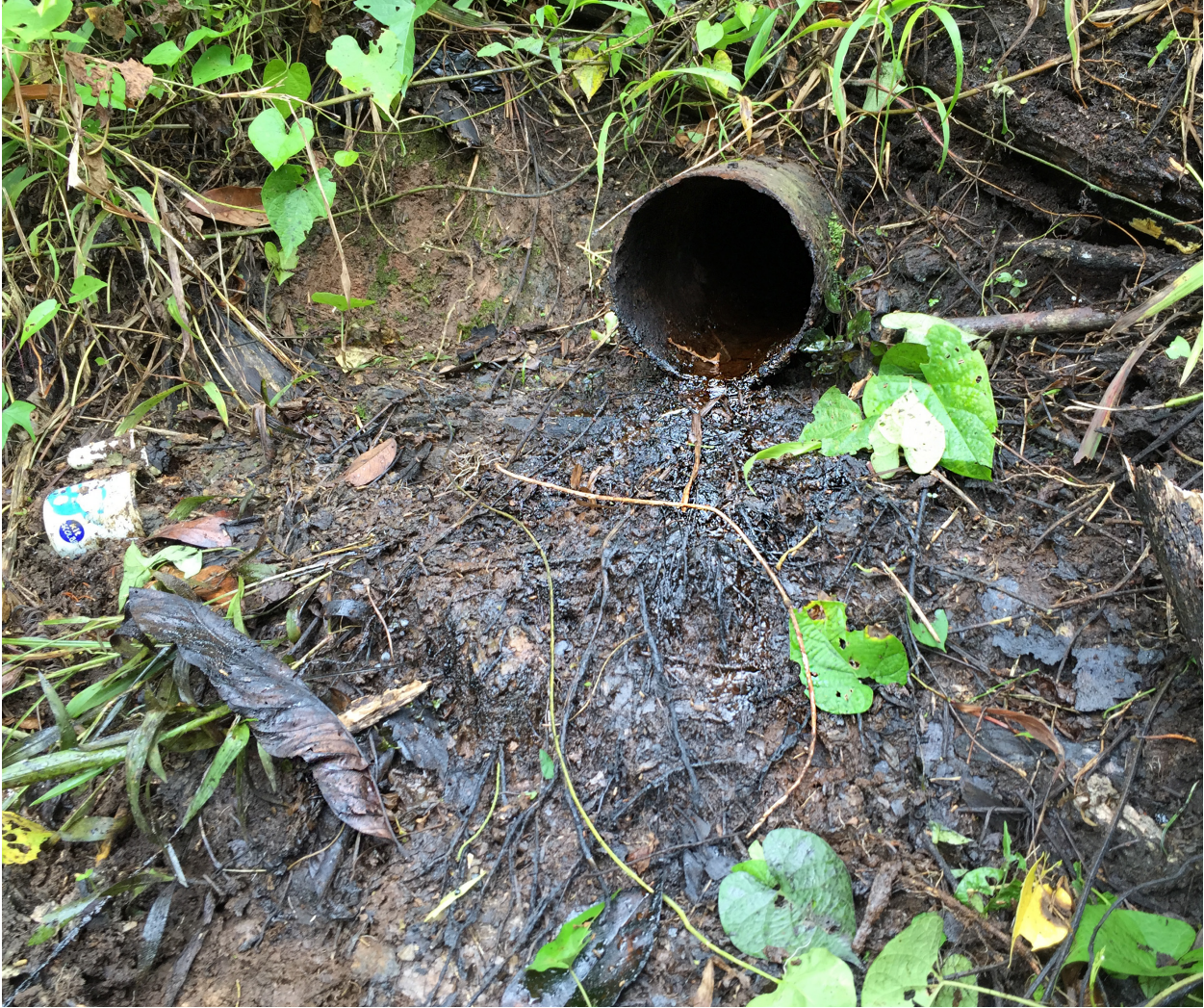
Lago Agrio 2, April 2015, crude extraction pipeline.
