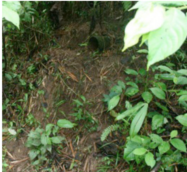
Drainage pipe beside Pit 3. The contaminated stream is located just below the pipe.
